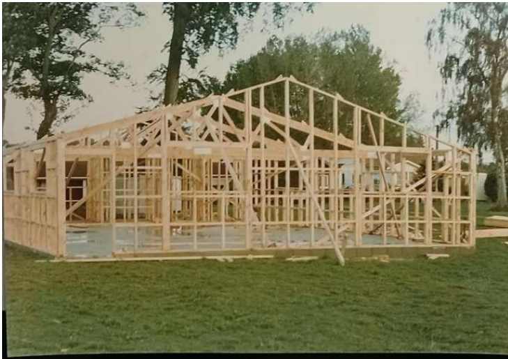
Rear view of the clubrooms under construction 1983
